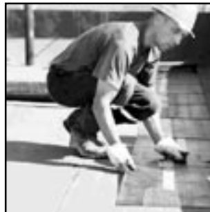
FLAT TOP ROOF
